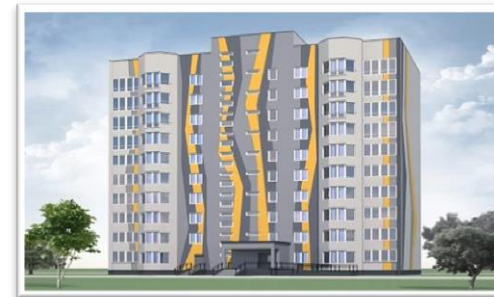
Housing construction in Kaluga
